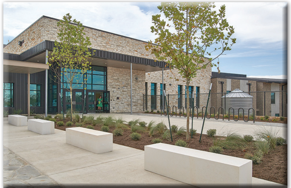
Dripping Springs Wildwood Springs Elementary School constructed by American Constructors
