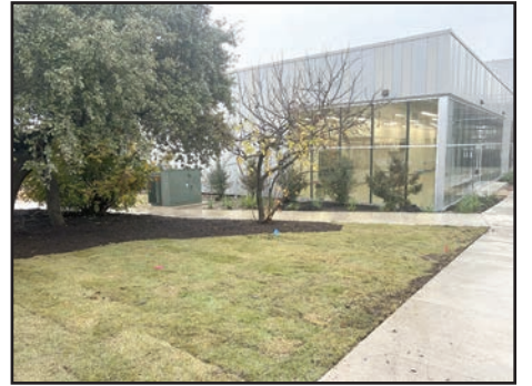
South Building exterior
