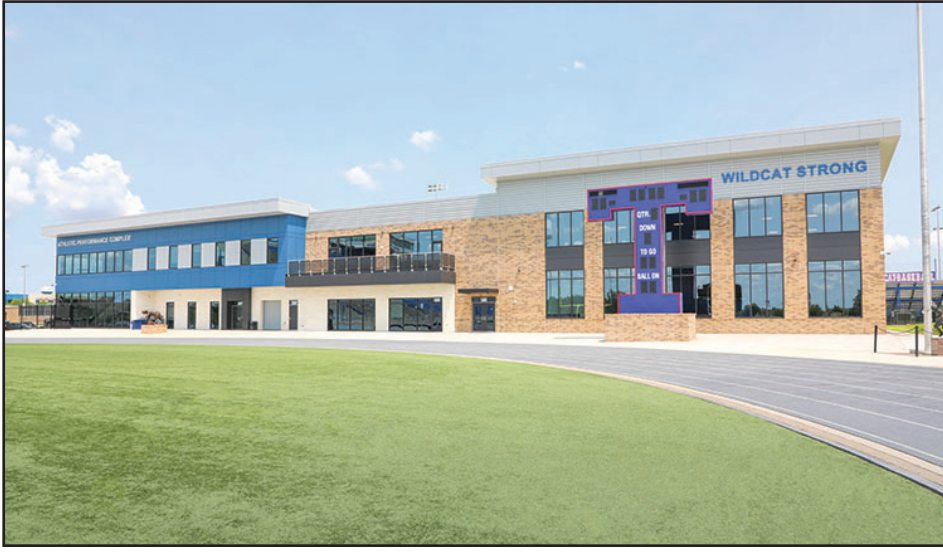
Temple Athletic Complex constructed by American Constructors
