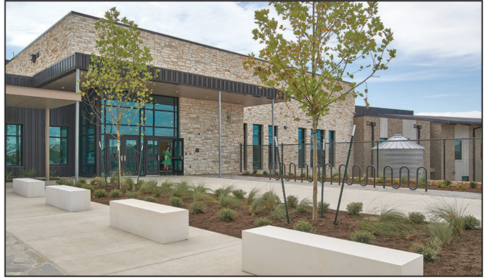
Dripping Springs Wildwood Springs Elementary School constructed by American Constructors
