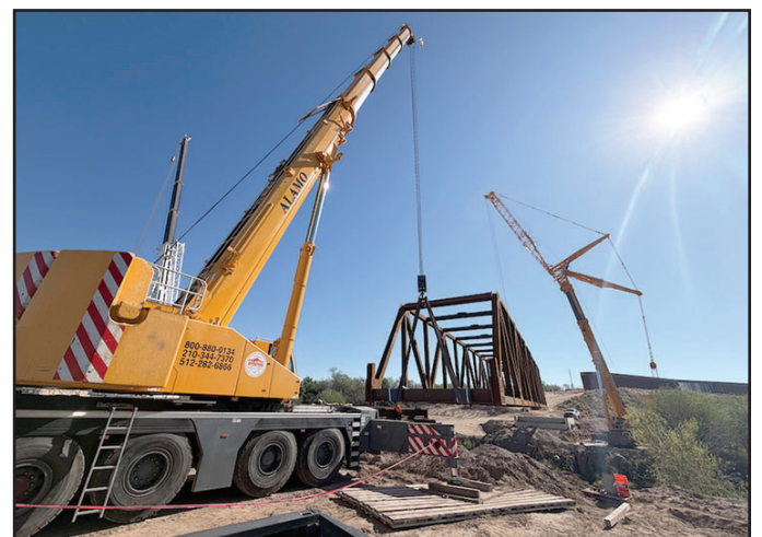
View of the bridge from Alamo Crane's LTM 1300-6.2, 360-ton Liebherr crane.
