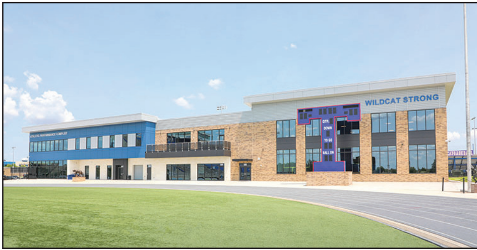
Temple Athletic Complex constructed by American Constructors
