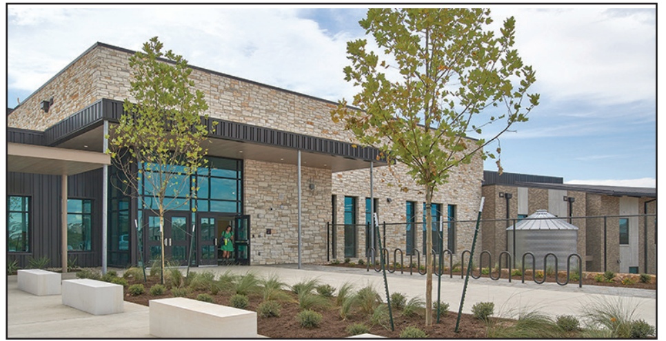
Dripping Springs Wildwood Springs Elementary School constructed by American Constructors
