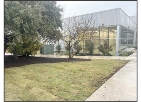
South Building exterior
