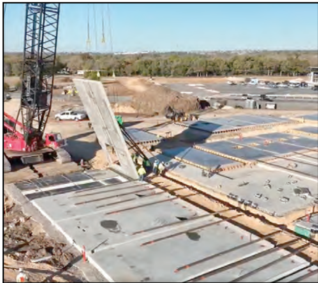
Construction continues on a new Austin-area headquarters facility being built by Structure Tone Southwest. The 9.5-acre ground-up project features concrete tilt-wall construction, structural steel, an interior mezzanine, a high-performance façade and extensive site infrastructure.
