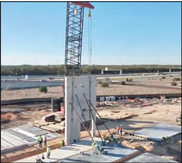
Construction continues on a new Austin-area headquarters facility being built by Structure Tone Southwest. The 9.5-acre ground-up project features concrete tilt-wall construction, structural steel, an interior mezzanine, a high-performance façade and extensive site infrastructure.
